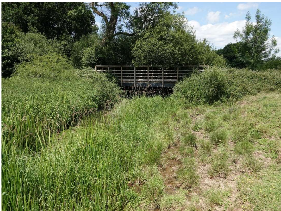
Overs Bridge and the Longford Stream on 18 June 2025
